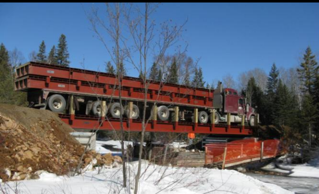
Photo 5: 18.3m Lessard Modular bridge crossing new Como Lake bridge enroute to Bass Lake (another MTO - Lessard Welding bridge project).
